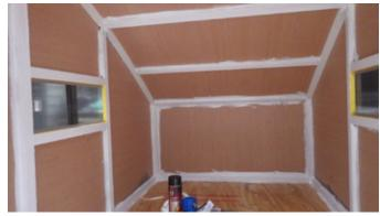
I started with a 4x8 trailer from Harbor Freight and shortened it 18 inches and added a plywood floor. I constructed the walls and framing from  $3/4 \ge 1-1/2$  pine and 1/4" underlayment. Everything was glued and screwed together. 3/4" thick foam sheets were glued to the inside walls for insulation.
