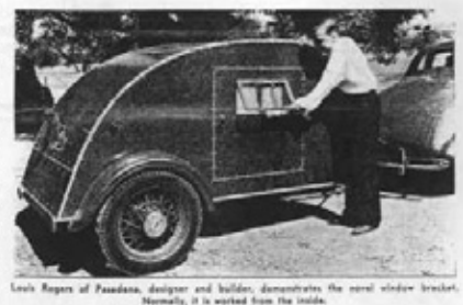
Louis Rogers of Pasadena, designer and builder, demonstrates the novel window bracket. Normally, it is worked from the inside.
