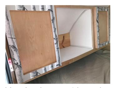
left over from a house project. I chose to only go with a small over head shelf on the front of the cabin and then a large cabinet with 2 doors and an opening for an a/c that will be installed in the future. The interior ceiling is sheets of shelf plastic and then covered with textured wallpaper.
