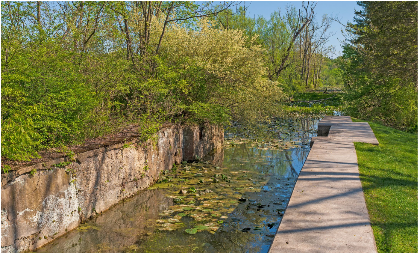
Lock remnant, Ohio & Erie Canal, Ohio
